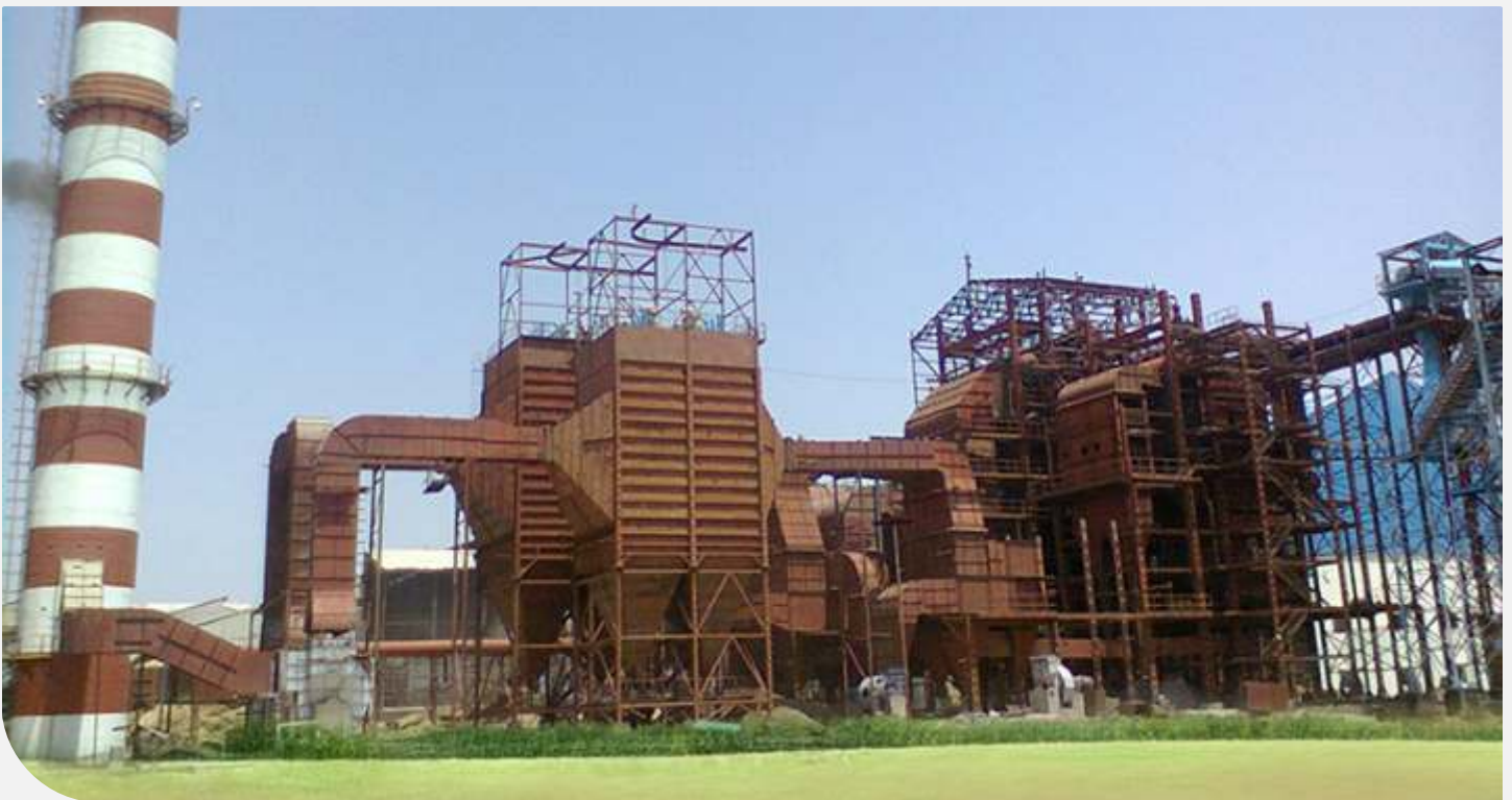
Vaidyanath SSK Ltd. 70 TPH, 87 Bar, 515°C 40 TPH, 87 Bar, 515°C
